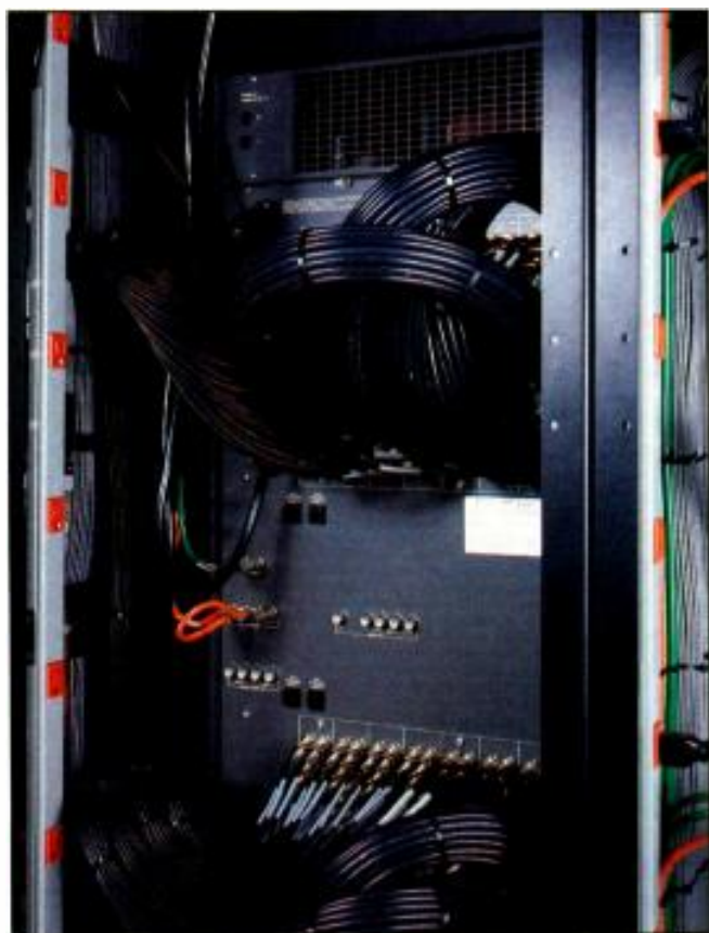
The original Belden 1694A 128x128 SDI Router cabling was reconnected and supplemented with the narrow diameter Belden 1855A for I/O 129-256.
